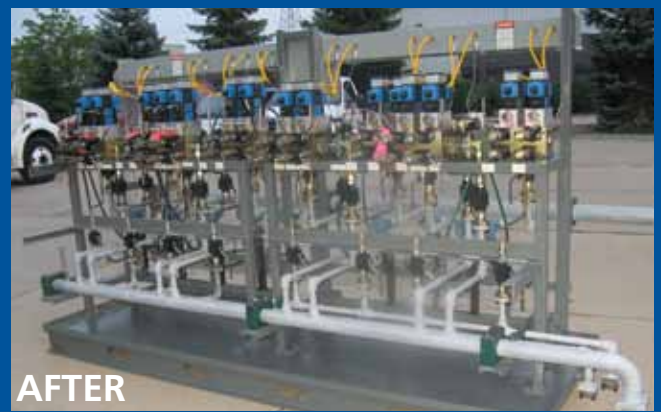
Valve Stand Rebuild
